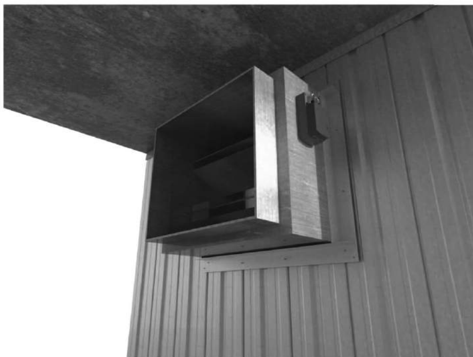
Figure 88 – Example of Damper Installation (duct not shown for clarity)
